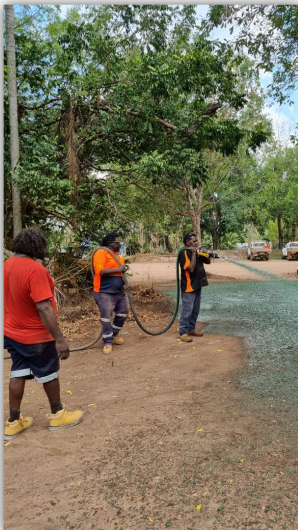
Hydro-mulching training for local workers supporting the new oval re-development, Ngukurr
